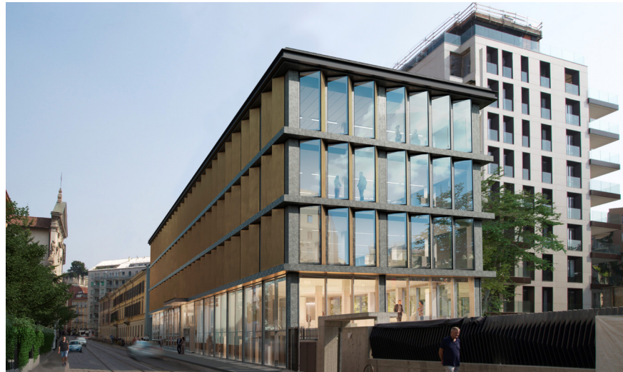
The project team retained the existing structure, fully reconstructing the interiors and adding a new facade.
